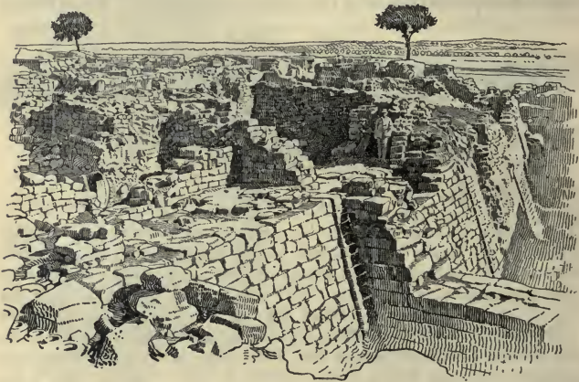
FIG. 63. THE WALLS OF HOMERIC TROY, BUILT ABOUT 1500 B.C.
